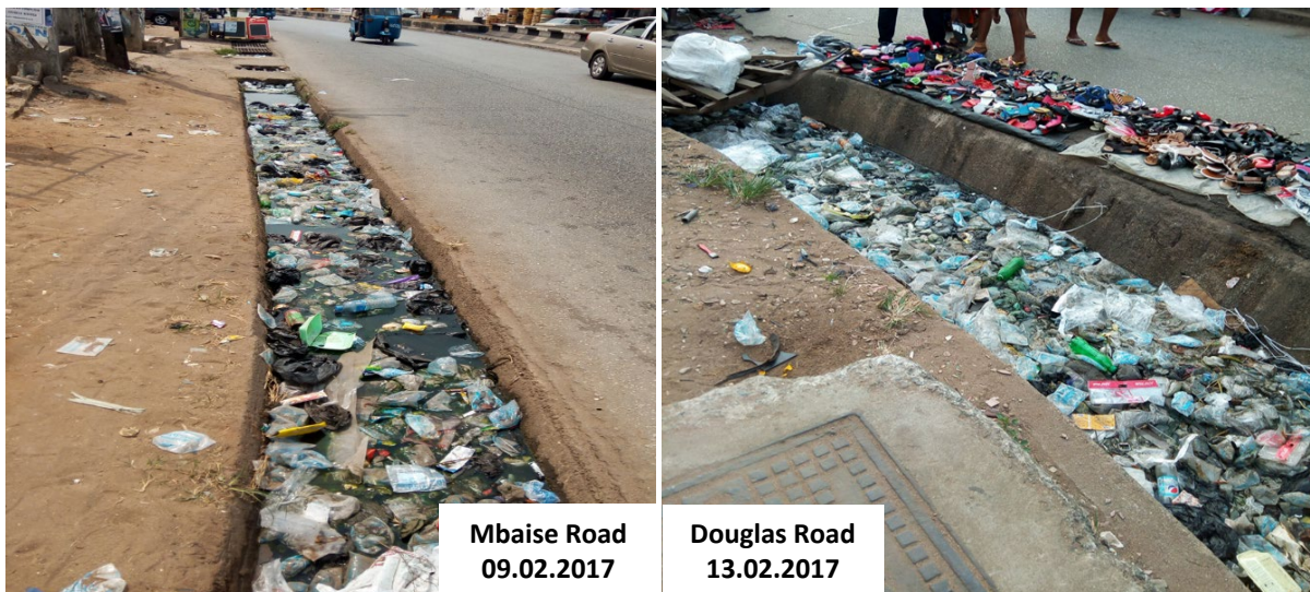
Figure 4.44c Examples of water channels in which Imolites dispose of used water. The photos were taken in the dry season; but the water channels are filled with stinking wastewater and waste. (Photos by Ache).
