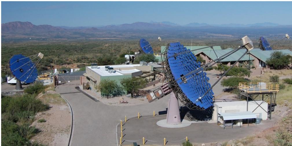
Figure 2.9: VERITAS. The Very Energetic Radiation Imaging Telescope Array System at the Fred Lawrence Whipple Observatory in south Arizona, consisting of four detectors. Image modified from [59].
