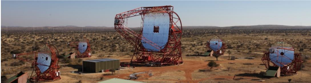
Figure 2.10: The H.E.S.S. telescope array. The four corner telescopes have a reflecting area of 108 m<sup>2</sup>, and the centre telescope has a reflecting area of 614 m<sup>2</sup> [62]. Image modified from [63].
