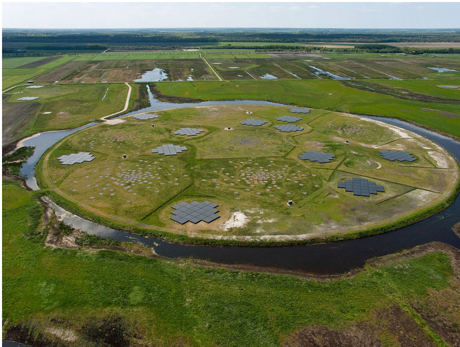
Figure 3.2: Aerial view of the Superterp, the densest array of stations in the ILT, located near Exloo in the Netherlands. The Superterp consists of six core stations with a maximum baseline of about 350 m. Credit: ASTRON/LOFAR
