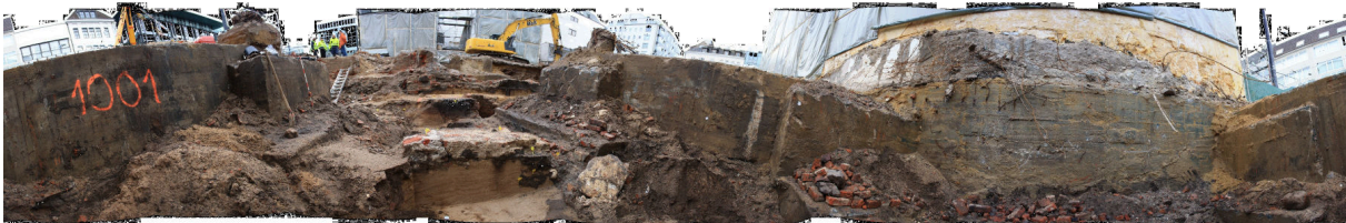
Figure 6.7: Panorama image of an excavation site.
