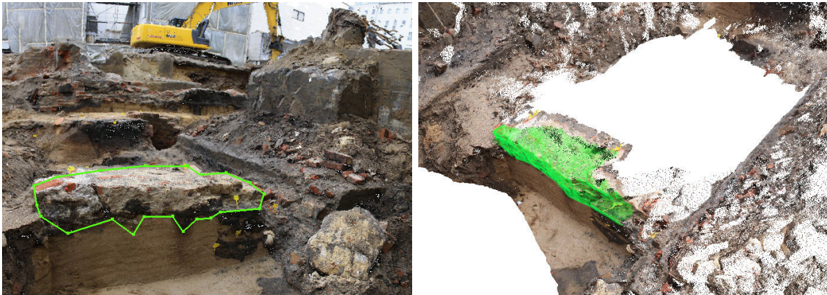
Figure 6.9: Left: 2D presentation of a selected region of interest in a point cloud. Right: 3D presentation of a selected region of interest in a point cloud.
