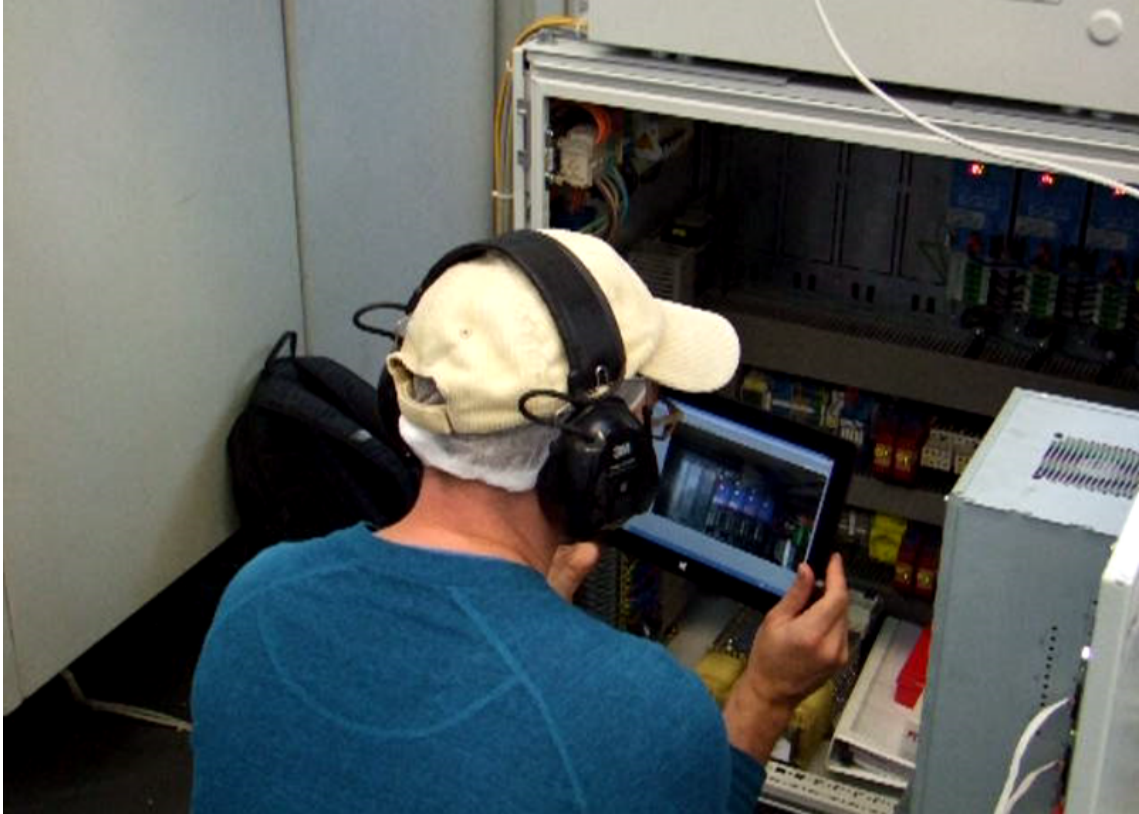
Figure 6.14: Test person with mobile device following the expert's instructions in front of the switch cabinet
