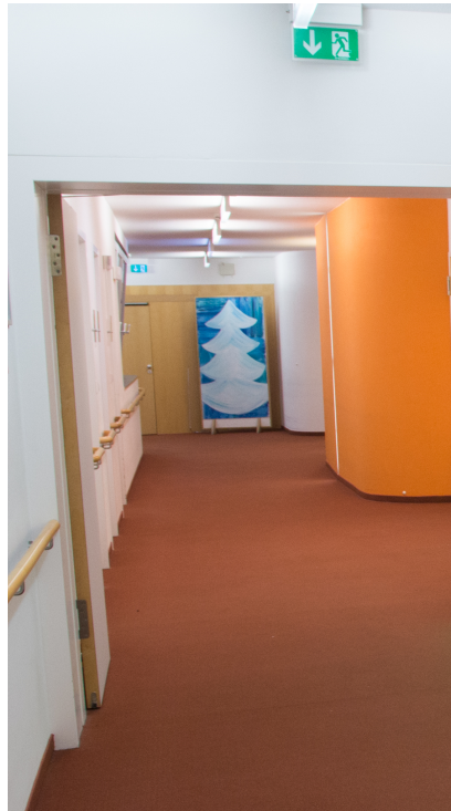
Fig. 5.2 Exit door in the facility D with the open button hidden behind a painting
