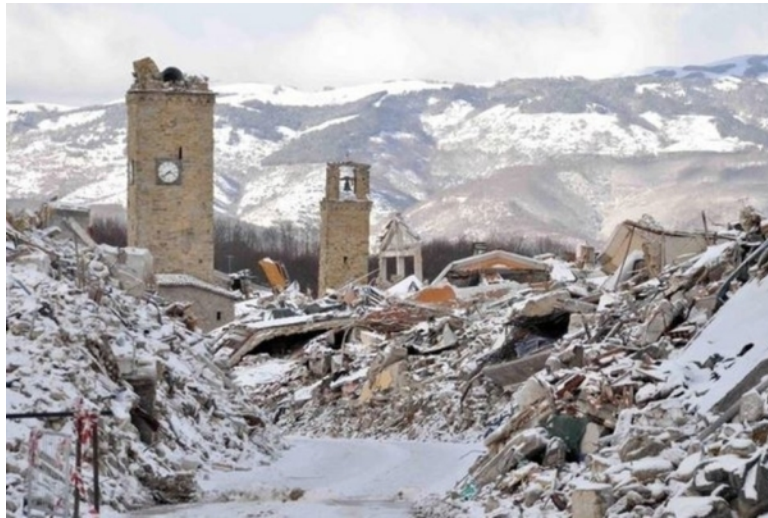
Figure 1.1: Disaster area of Amatrice in Italy after the earthquake on 18th January 2017. [20minuten.ch, 2017]
