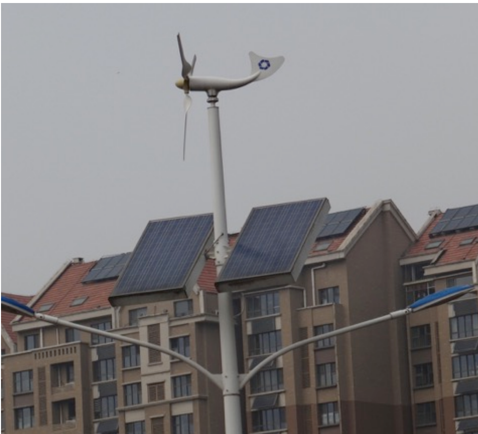
Figure 10: Solar Panels on the Street Lights and Roof Tops in the SSTECH
