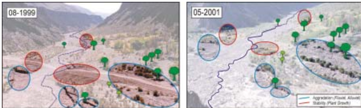
Fig. 184 and 185: Examples of present fluvial dynamics and floodplain modifications in the Quebrada de Purmamarca close to Lipán. Note the tendency to aggradation in the river bed and aggradation by debris-flow / alluvial fan activity (large blue circle); aggradational tendency does not seem to be restricted to the valley floor.
