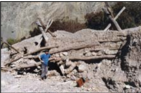
Fig. 188: Wooden fence on the floodplain at Purmamarca to divert debris-flows and flooding and prevent overflowing into village.
