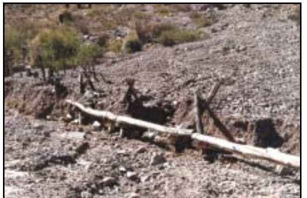
Fig. 189: Wooden fence of similar construction as Fig. 188 at Lipán. Note amount of burial the fence has experienced by a single debris-flow event in 1999.
