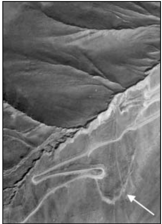
Fig. 111: Scar of possible future landslide in the upper Quebrada de Potrerillos (GASATACAMA aerial photography, image width ~700 m).
