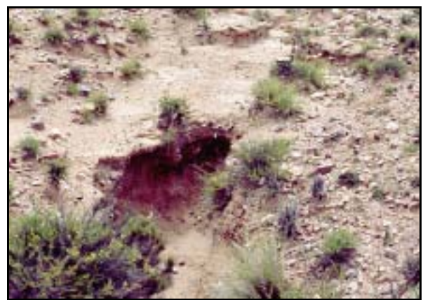
Fig. 67: Gully headcut on top of terrace T-3 at Lipán. Note distinct soil horizon of high erosional resistivity.
