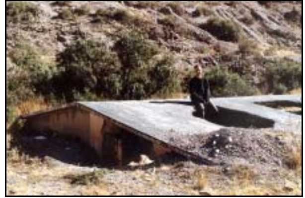
Fig. 187: Building of the former railway station of Purmamarca in the Quebrada de Humahumaca which was buried by a single debris-flow event in 1984.
