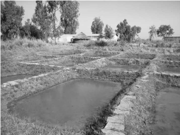
Fig. 4: Ponds after plantation of the dams and their protection with flagstones. The store-hut is visible in the background.
