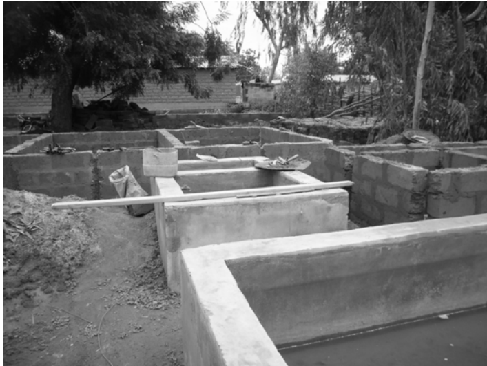
Fig. 1: Newly constructed catfish-nursery in Malanville
