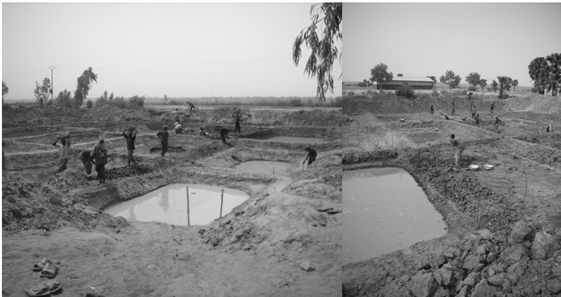
Fig. 3: Manual digging of the 15 experimental ponds
