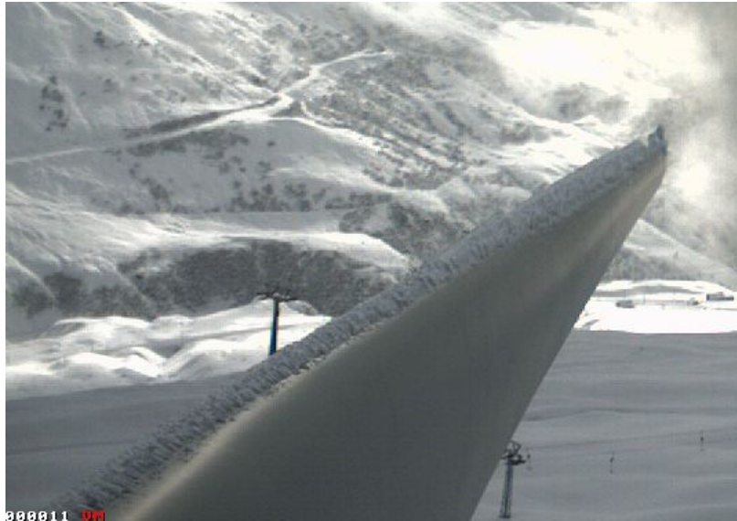
Figure 3: Ice accretion on the blade of a wind turbine (photo: CATTIN 2008)
