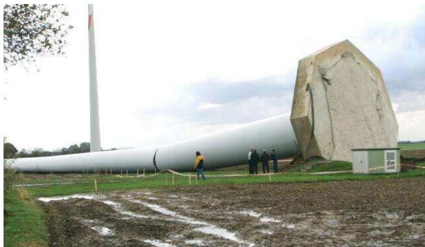
Figure 5: Complete failure of a wind turbine pole (photo: GEGENWIND SH)
