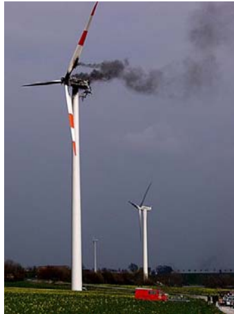
Figure 7: Burn down of a wind turbine. Black smoke comes out of the nacelle. The reason for the damage is not known (photo: ©GESAMTVERBAND DER DEUTSCHEN VERSICHERUNGSWIRTSCHAFT)
