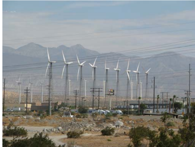
Figure 11: Lattice steel masts for wind turbines (photo: SIEBER 2011)
