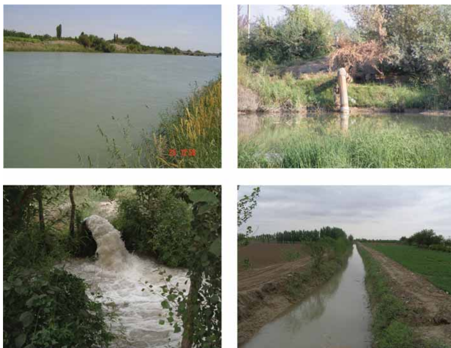
Figure 2.8: Some features of the irrigation system in Khorezm. The water is regionally distributed via irrigation canals of different sizes (upper left). Pumps are used to lift water to a higher level (upper right). From there it is distributed to farmers' fields via a huge network of smaller canals (lower left and right).
